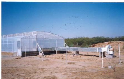
Figure-1: Fully Furnished Greenhouse, Kothara-Kutch Showing Blower and Suction Duct
