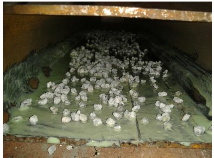
Fig: Application of epoxy and M- sand particles
