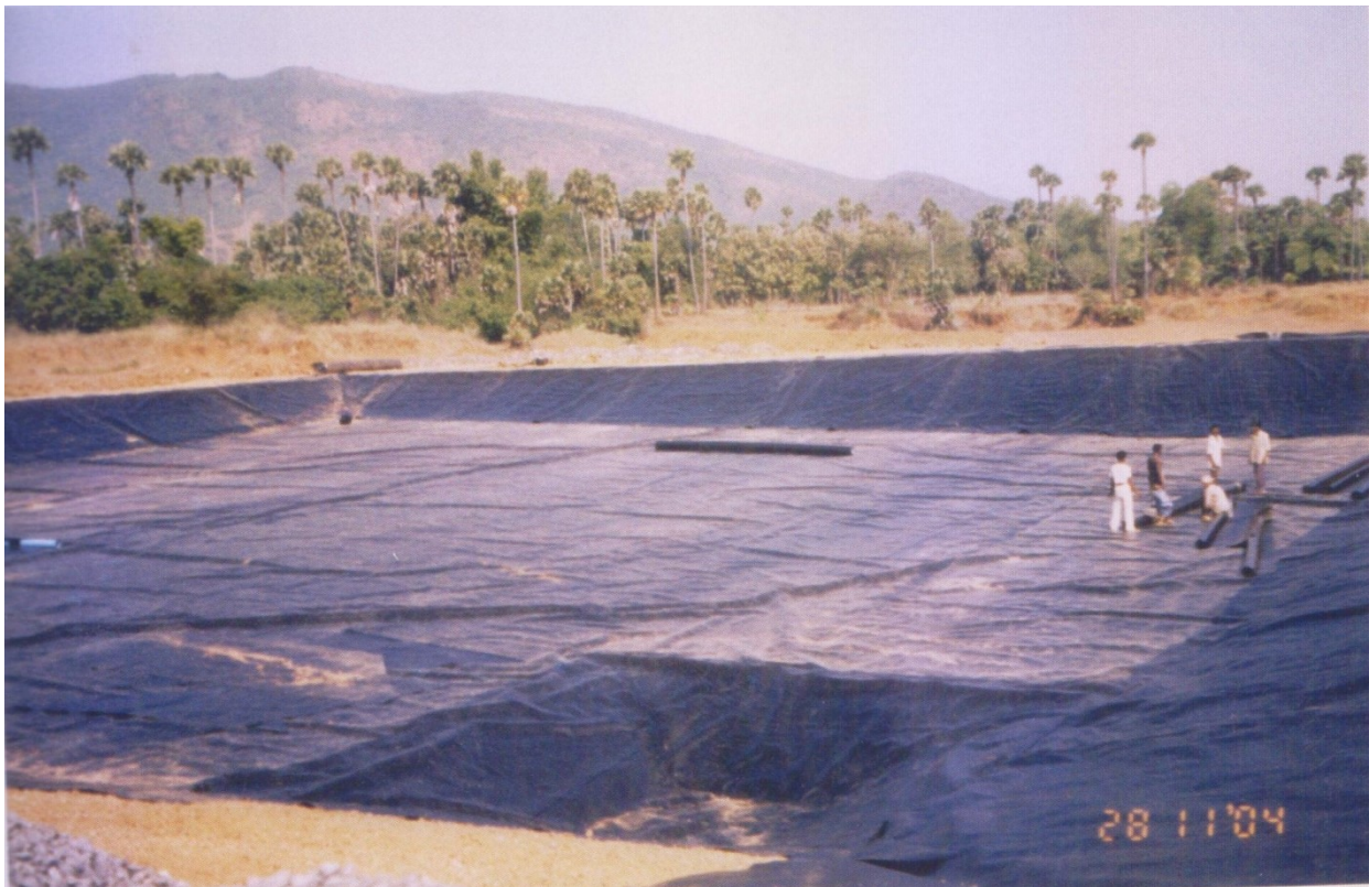
Figure 2. A view of Landfill with HDPE Geo-membrane
