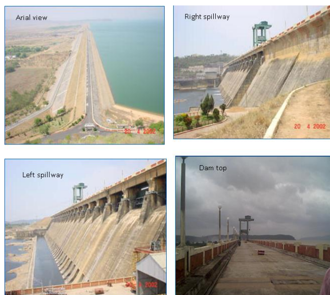
Figure 1. Views of the Hirakud Dam across the river Mahanadi, Odisha
