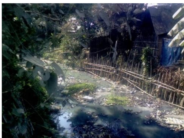
Figure 2. Impediment in the drainage system
