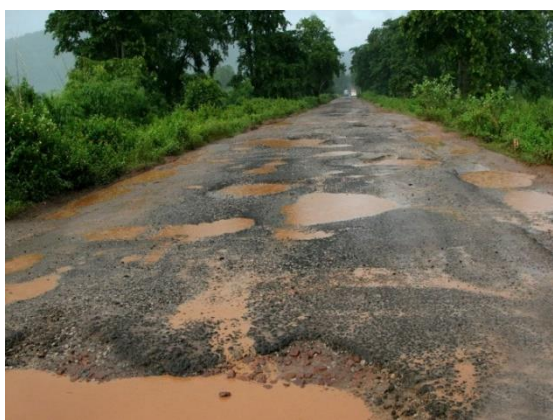
Fig. 1. State of roads with potholes
