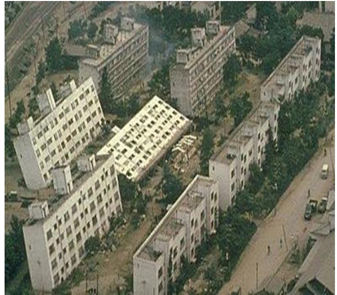
Fig.1.1 Failure of multistoried buildings during Niigata earthquake (1964), a city located on Sad island, in the Chūbu region of Japan.
