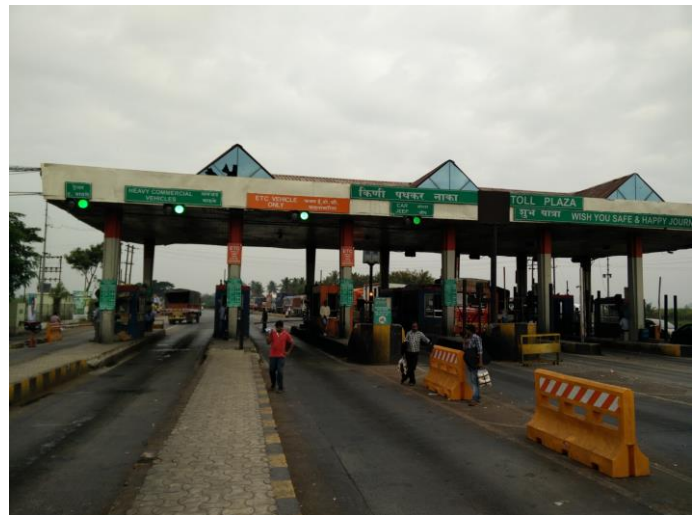
Figure 1: ETC at Kini toll plaza (Maharashtra, India)
