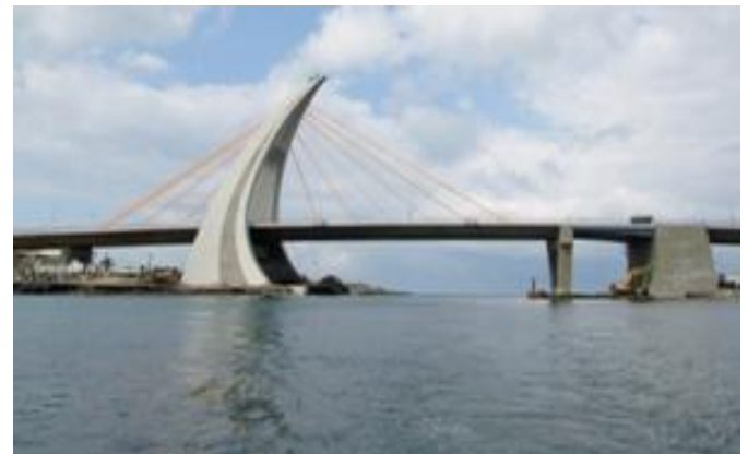
Figure 7: Outward appearance of the case bridge (close gate)
