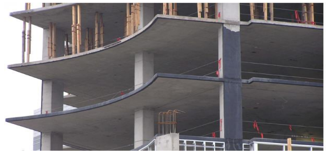
Figure 1 : Flat Plate Reinforced Concrete Structure
