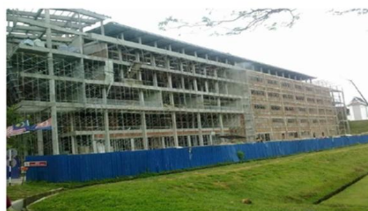
Figure 4: Construction in faculty of Electrical Engineering
