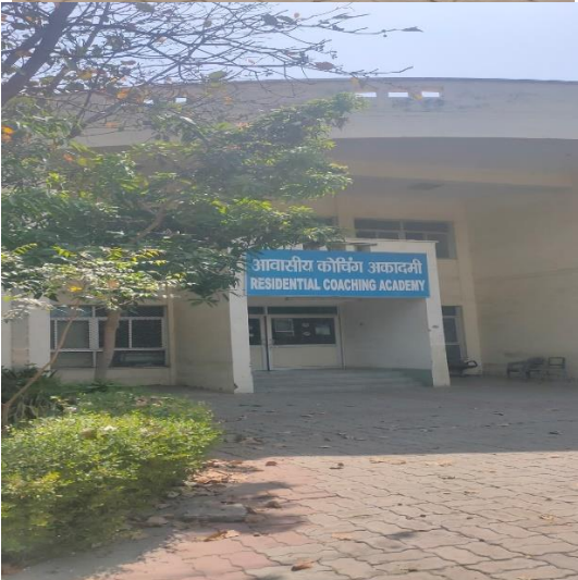
Boys Hostel : The coordinate of location for the boy's hostel building is X : 26.770839 and Y : 80.919419
