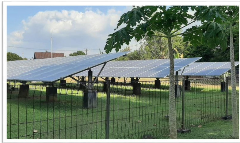
Figure 8: Photo of Tree Shadows on Array Surface 4
