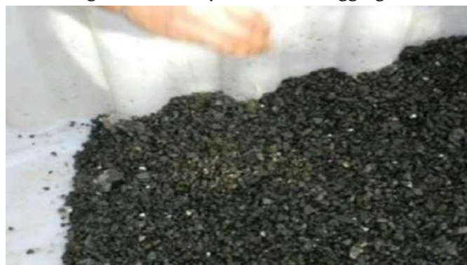
Fig 3 : Third layer of 10 mm and 5 mm aggregate
