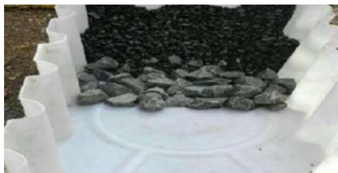
Fig 2 : Second layer of 20 mm aggregate
