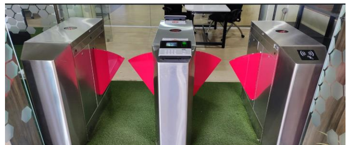
Fig 3. Security with RFID Gates and biometric attendance at MRUH.
