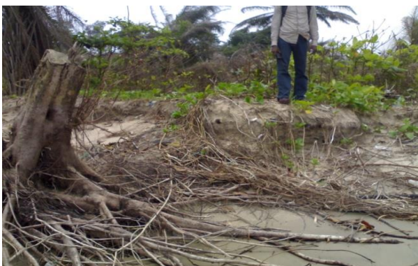
Plate 8 Photo at transect 8 (T8) showing active erosion site
