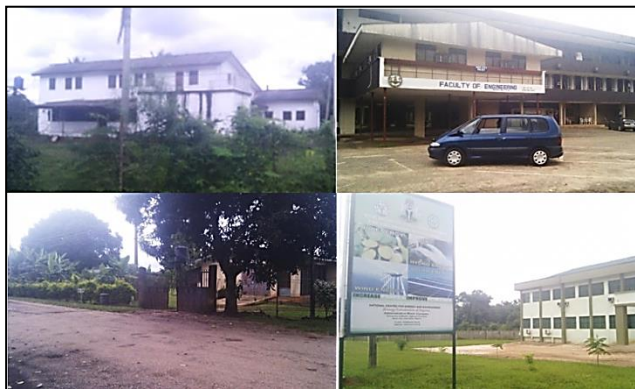
Plate 2: Sample photo views of the mapped buildings (Source: fieldwork, 2014)
