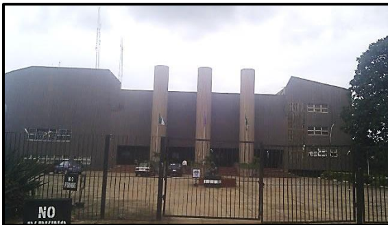
Plate 3: Façade photo view of auditorium
