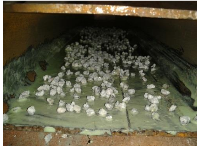
Figure 4 : Application of epoxy and M- sand particles
