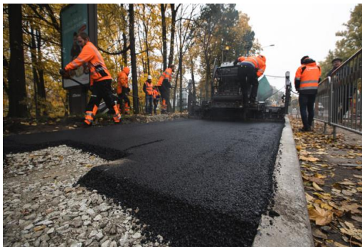
Figure: 8 Mixing of plastic, bitumen and aggregate
