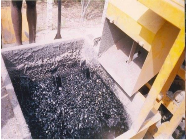
Figure: 6 Heating of bitumen
