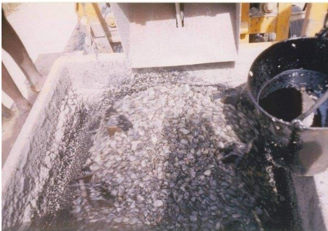
Figure: 7 Shredded plastic with hot bitumen
