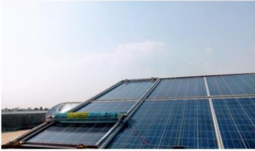
Figure 4 : solar panel cleaning using roller brush.
