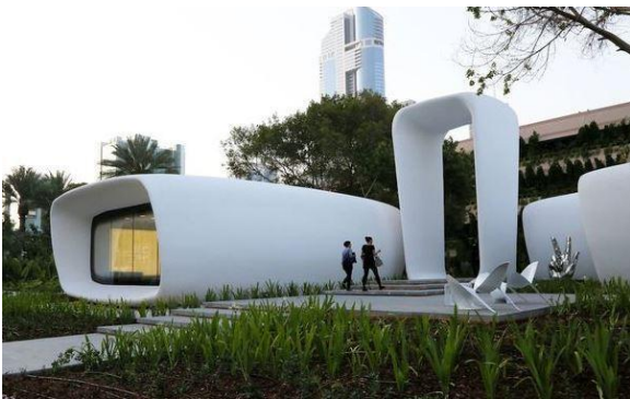
Fig 1 : 3D concrete printed office in Dubai, UAE
