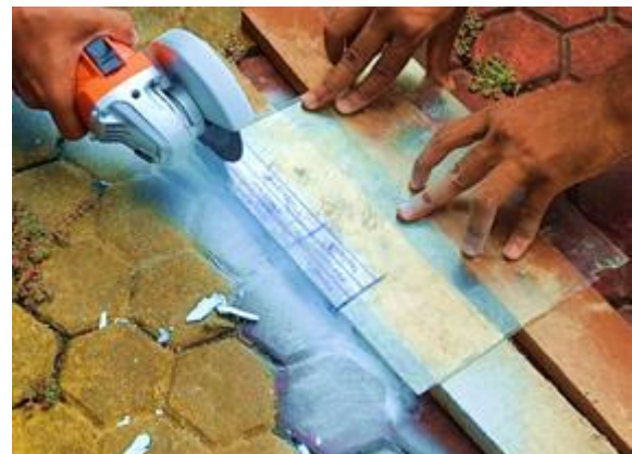
Fig 2.2 Cutting the slabs to the dimension
