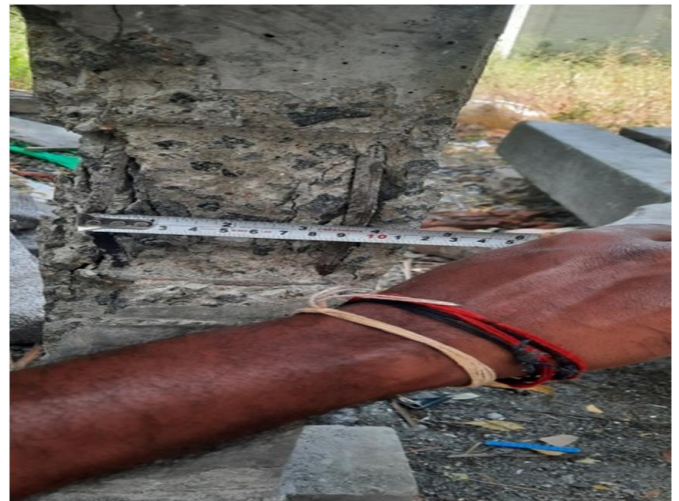
Fig. 4 Buckling of column
