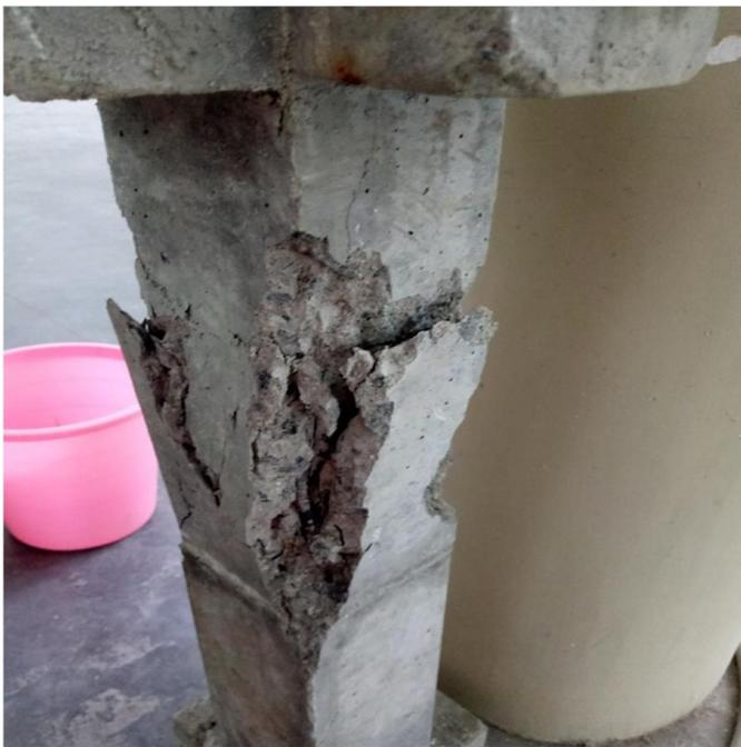
**Fig.6 Buckling Of Column**
