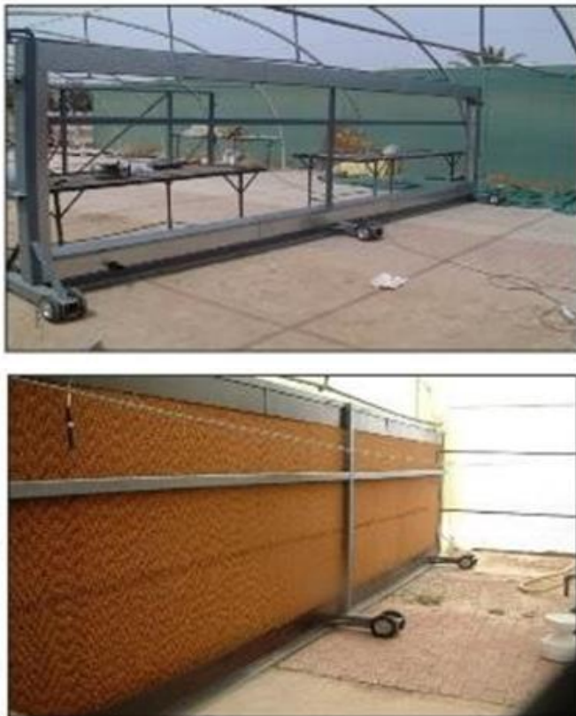
Figure 1. Moving frame mounted on wheels for the second wall of evaporative cooling pads
