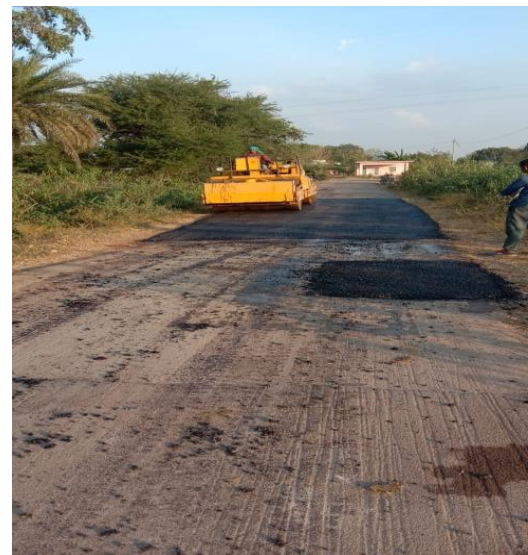
Fig 2.6 Repaired Potholes
