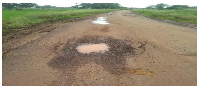
Figure 2.1 : Identified potholes
