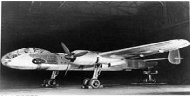
Ju 288 V1 first prototype, showing its complex "folding" main undercarriage.
