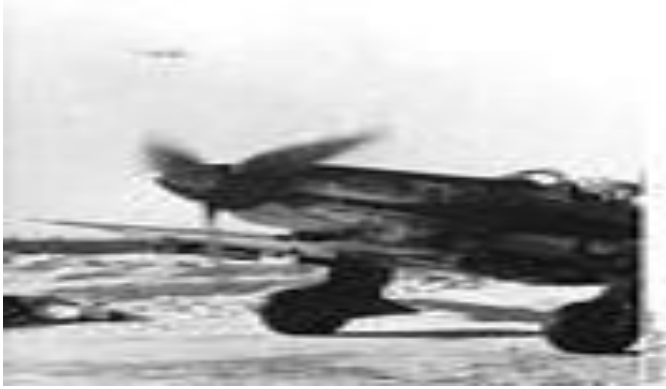
A Ju 87D with a wheel spat on its right wheel, absent on its left
