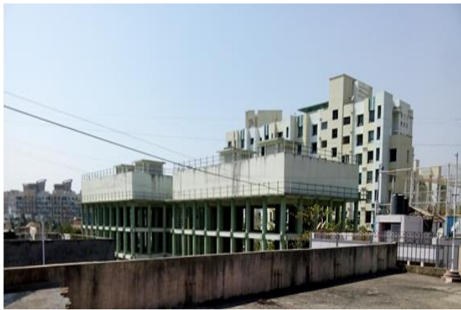
Fig 4 : Huge Municipal water storage tank on eastern side
