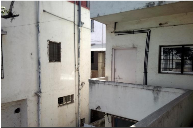
Figure 3: Abutting G+2 residential building on north side
