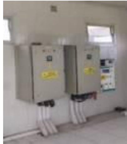
Figure 22. AC Distribution Side Condition of PV Power Plant 3 Source: PLN UIW Maluku, 3/4/2022
