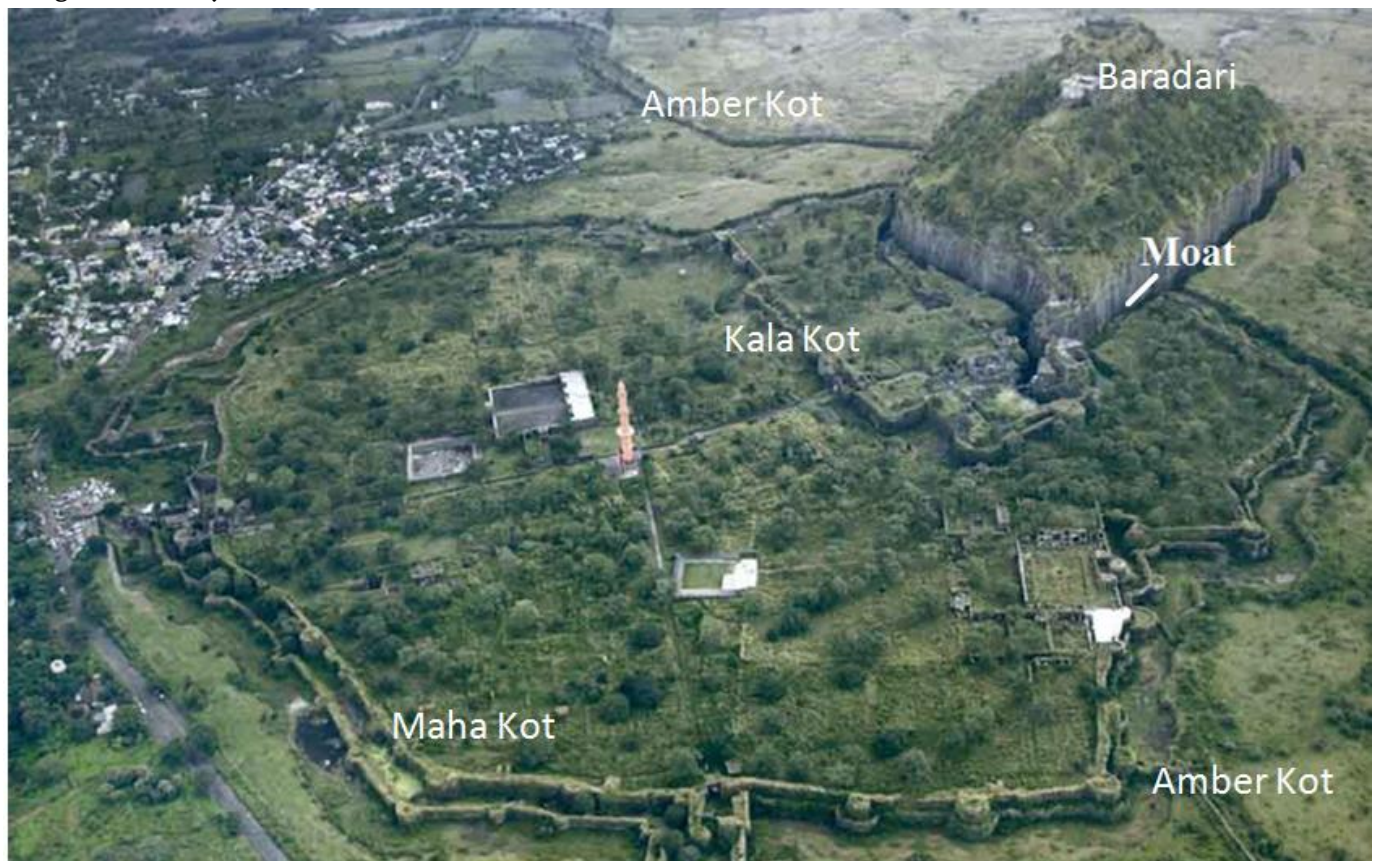
Fig 2 : Fortification walls dividing the fort area
