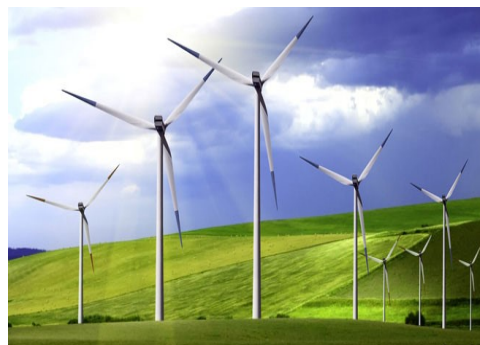
Wind mill as an energy resource
