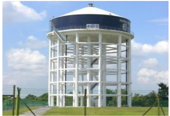
Fig: Intz type water tank
