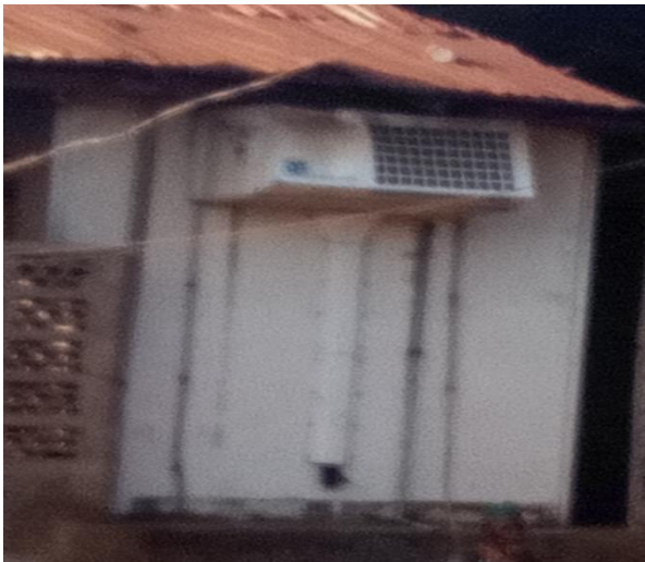
Figure 6. Sample of Private Cold-room at Durbar Area, Oyo East L.G.A.
