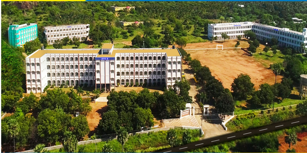
Aerial View of AVCE
