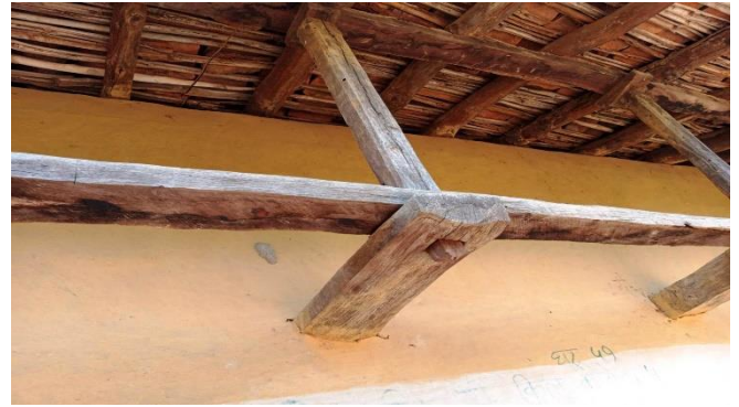
Fig 4 : Structural simplicity of overhangings
