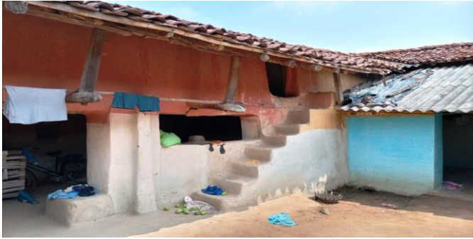
Fig 2 : Staircase constructed with mud blocks leading to attic
