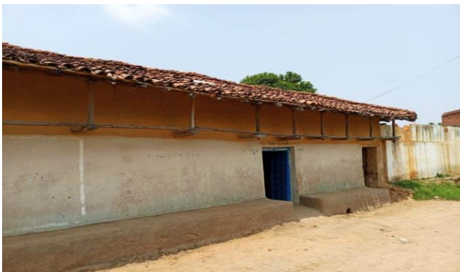
Fig 3: Wall protection by overhanging roofs
